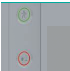
Buttons located in the door frame to activate the door in different modes
